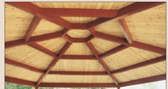
Tongue & Groove (T&G) Roof Interior
