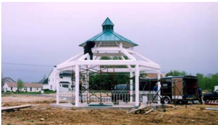
The upper metal panel roofing is installed, then the cupola For multi-rib roofing, all panels are factory cut
