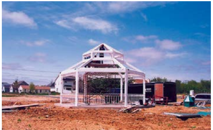
Frame complete and ready for roofing
