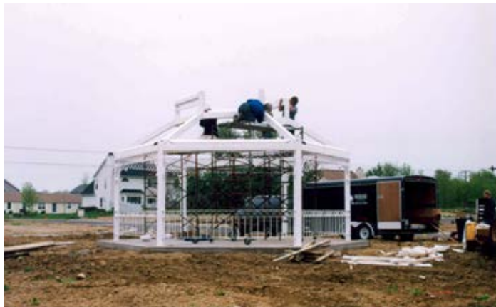
Railing & ornamentation are installed with the frame
