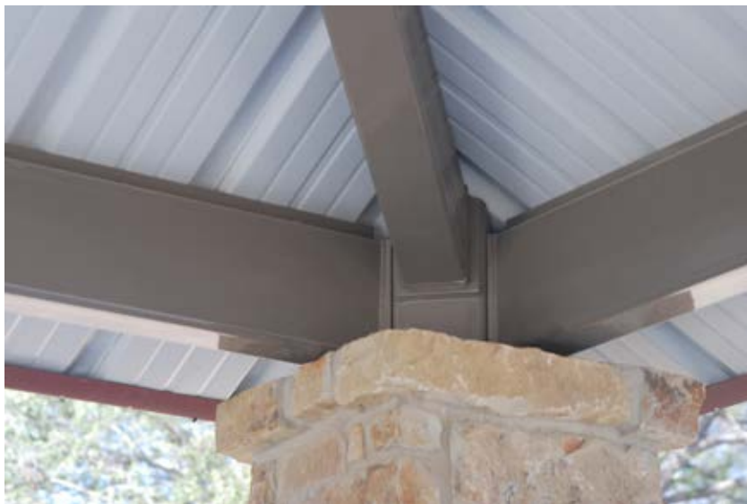
Connection Detail (Typical frame detail for square model)
