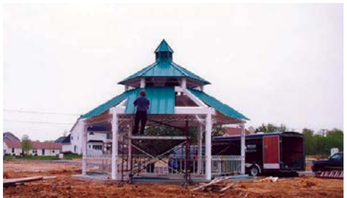
Installation of lower roofing panels
