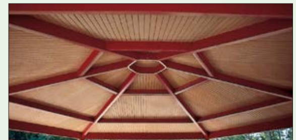
Structural Insulated Panel (SIP) Roof Interior
