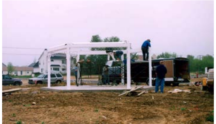
No field welding required during erection
