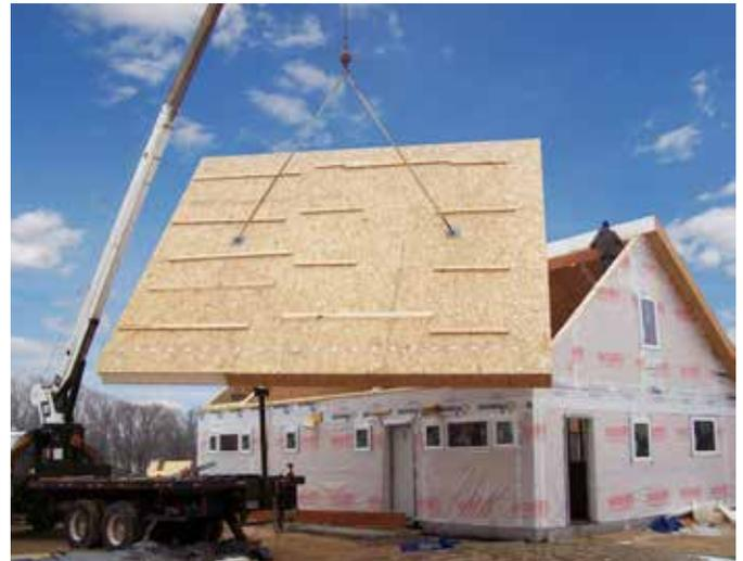
Large panels assembled on the ground, then lifted.
