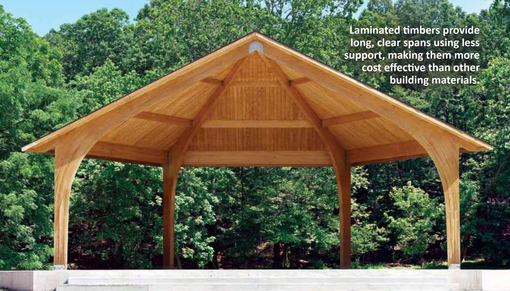
Laminated timbers provide long, clear spans using less support, making them more cost effective than other building materials.
